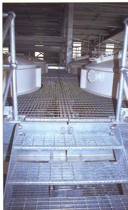
BOLTED fixing, Holed end plates, Abrasive nosing.
